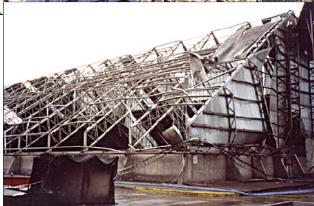
The Toepfer Puerto San Martín explosion in Santa Fe, Argentina in 2001 started with a primary explosion that caused chain-reaction second and third explosions.
