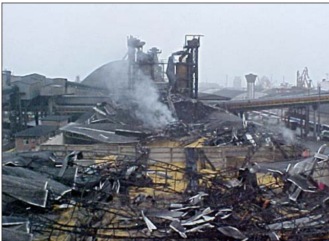
The 2001 Coinbra Paranagu  Terminal explosion in Paran , Brazil, blew five-ton pieces of concrete 300 meters, and grain continued to burn for nearly three weeks.
