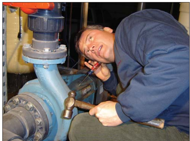
The UE Ultraprobe 10,000, left, can detect bearing failures in the very early stages of failure. In the photo on the right, you can see the predictive technique used in the 1970s for detecting bearing failures, and possibly the fault correction tool.
