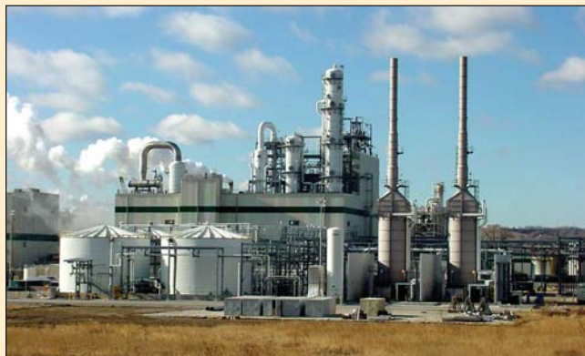
The PLA manufacturing plant in Blair, Nebraska.
