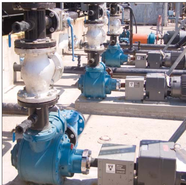
Throughout its biodiesel plant, Peter Cremer North America, LP uses NP2 or NP4 sliding vane pumps manufactured by Blackmer, Grand Rapids, Michigan.
