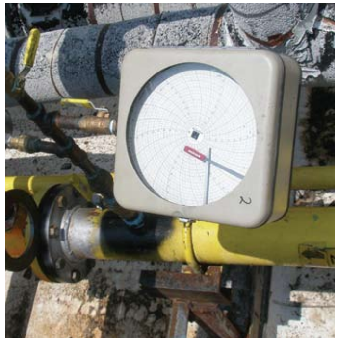
Fig. 4: A pressure chart recorder
